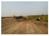
Aug 10/18 Workers installing silt fence around water course crossing
